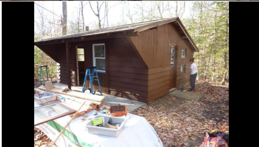
Cabin renovation progress – November 2016 (Photos courtesy of Range Dave)
